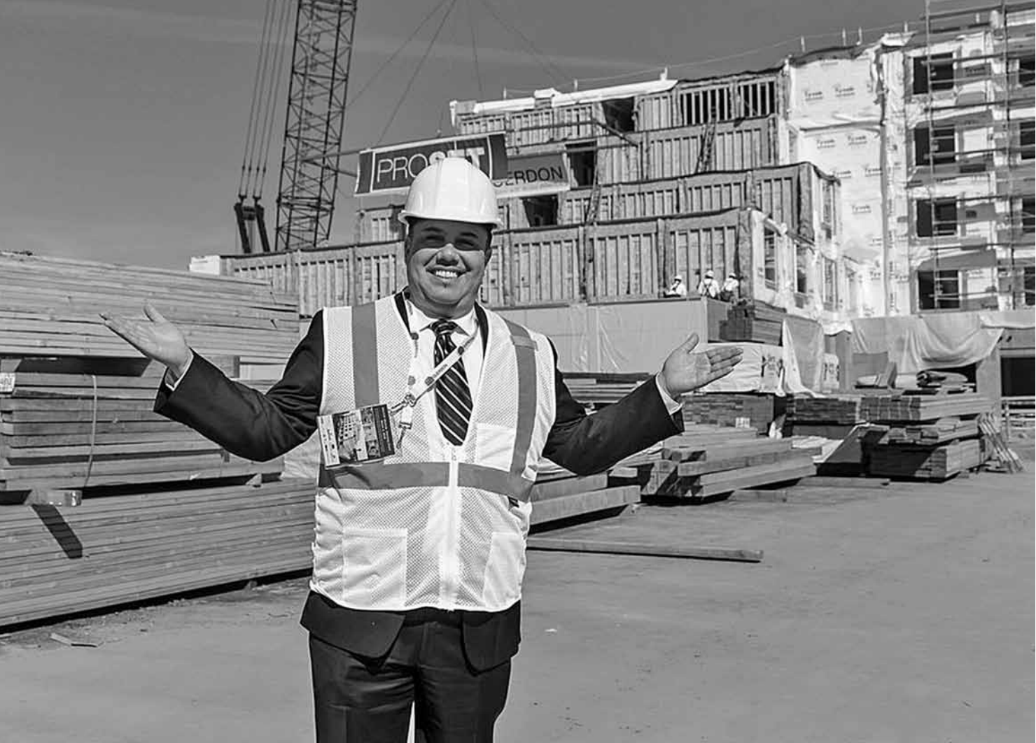
The Marriott Modular Stacking Event took place on March 6 with the Courtyard and TownePlace Suites Hawthorne representing the first dual-branded project in the Marriot Modular Program. A crowd of more than 300 hotel developers, architects, investors and civic leaders (including Mayor Alex Vargas shown in the photo) gathered at the 4.2-acre site across from City Hall and watched a crane hoist some of the last remaining rooms atop the five-story development, which resembles a giant set of building blocks. Photo by Erick Chavez.
