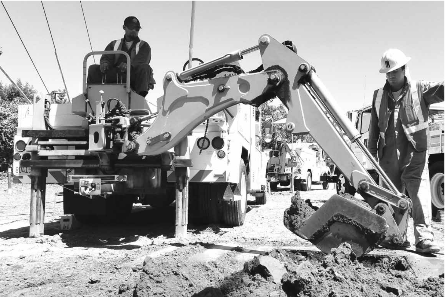
A lead construction technician learns how to operate a backhoe at Situation City, a training facility in Los Angeles. The training is designed to prepare construction technicians to respond and repair natural gas lines that are damaged by dig-ins out in the community. Photo provided by SoCalGas
