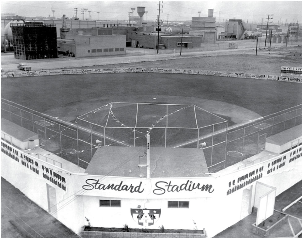
The year 1961 was the inaugural season for Standard Stadium, home of El Segundo American Little League. This baseball stadium was built by volunteer dads from El Segundo American Little League and was played on until 1979 or so. The stadium was located on Mariposa Avenue where the U.S. Post Office currently stands. Duley Road runs along the outfield to the east. Photo provided by Julie Stolnack.
