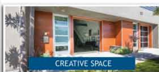
CREATIVE SPACE 219 California Street Fully equipped office condominium is set on a one acre site and has 6 parking spaces.
