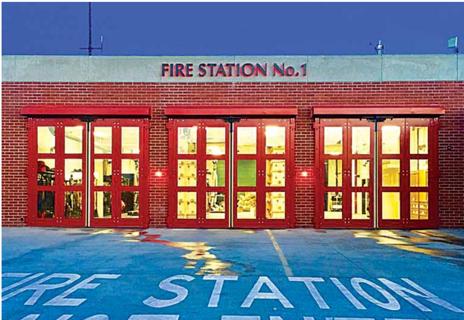
The crews from Engine-31 and Rescue Ambulance-31 recently returned to the bolstered Fire Station 1 on Main Street. They were displaced due to a significant remodel and earthquake retrofit project that is now complete. Photo Courtesy of El Segundo Fire Department.
