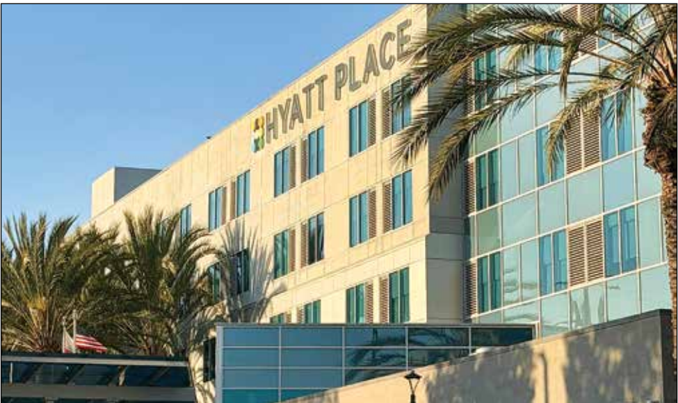
An AI data center was proposed on the site of The Hyatt Place hotel in El Segundo. The developer unexpectedly abandoned the project during a July 9 public hearing that drew a large crowd of residents and neighbors to the east of El Segundo opposed to the plan. Photo by Stella Cordova.
