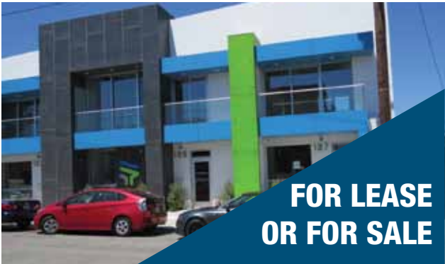
127 - 129 LOMITA ST BRAND NEW CONSTRUCTION 3,600 SF
