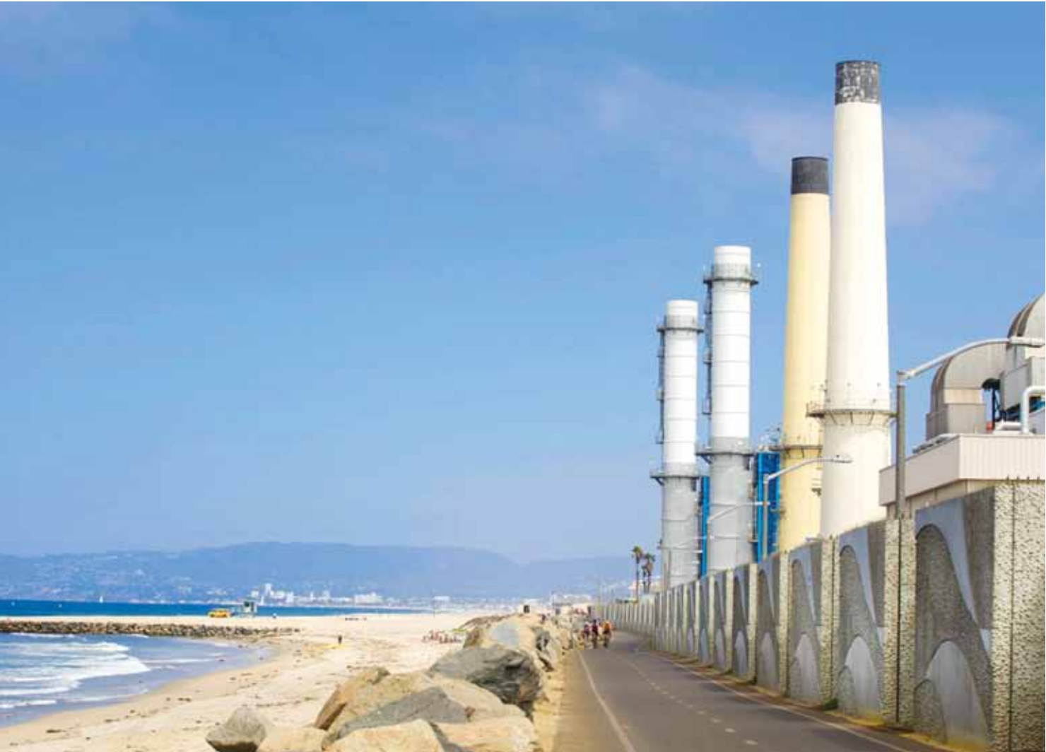
A view of the El Segundo Beach bike path, facing north. The right-side retaining wall was built to protect the NRG plant from large ocean swells. Photo by Peter Thornton. ♦
