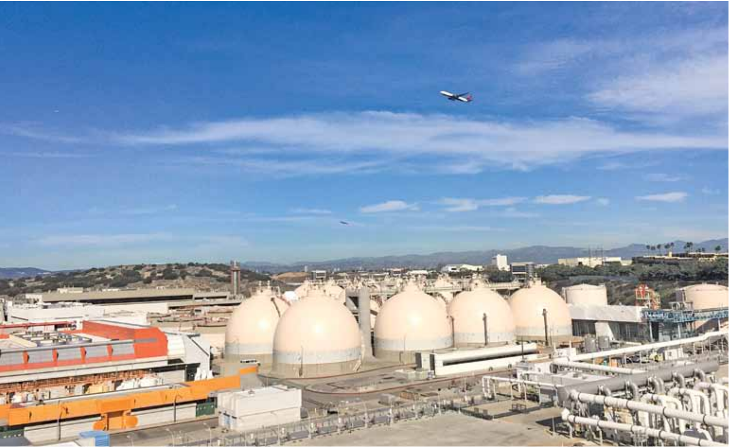
A bird's-eye view of the Hyperion Plant in El Segundo. The plant has been in operation since 1894, although it has been extensively renovated many times, the first time in 1950. Photo by Peter Thornton, jp.thornton58@gmail.com. ♦
