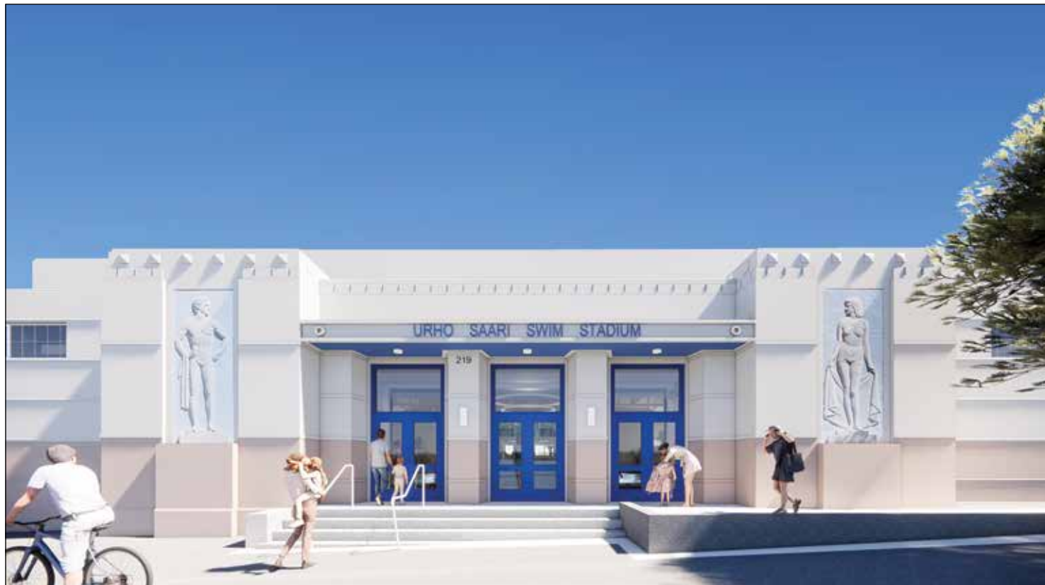
The refreshed Plunge design maintains its historic character and iconic Art Deco facade while renovating the interior to meet today's building standards. Photos provided by the City of El Segundo.
