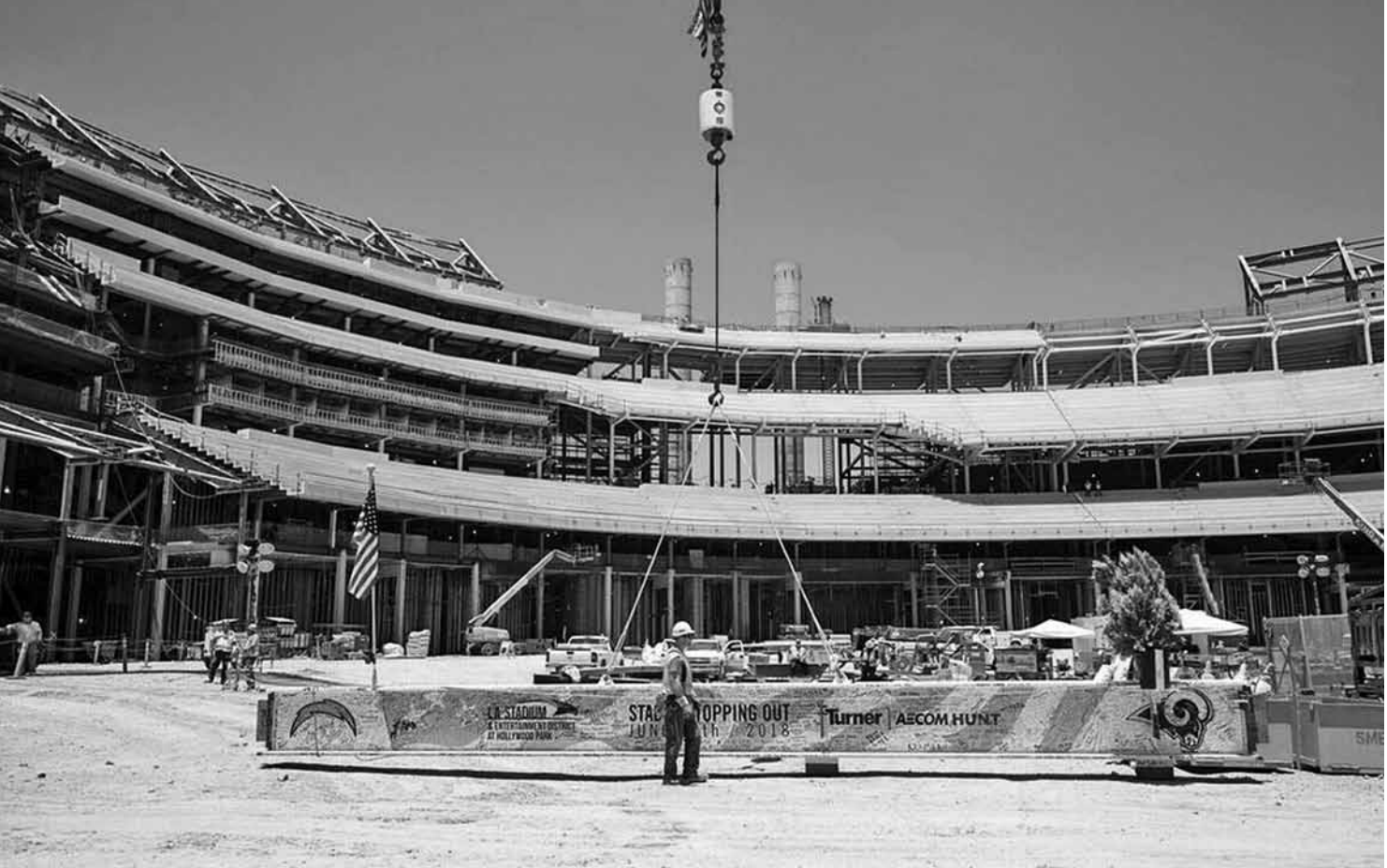
Last week was the topping out ceremony for the LA Stadium commemorating the placement of the highest steel beam on the structure. Inglewood Mayor James T. Butts, project principals and LA Rams and Chargers officials were among those in attendance. The final beam for the stadium bowl is 42 feet long and weighs 12,000 pounds. Tradition calls for an evergreen tree to be placed on the beam to symbolize good fortune, continued growth and a safe work environment. Photo by Hiro Ueno, LASED. •
