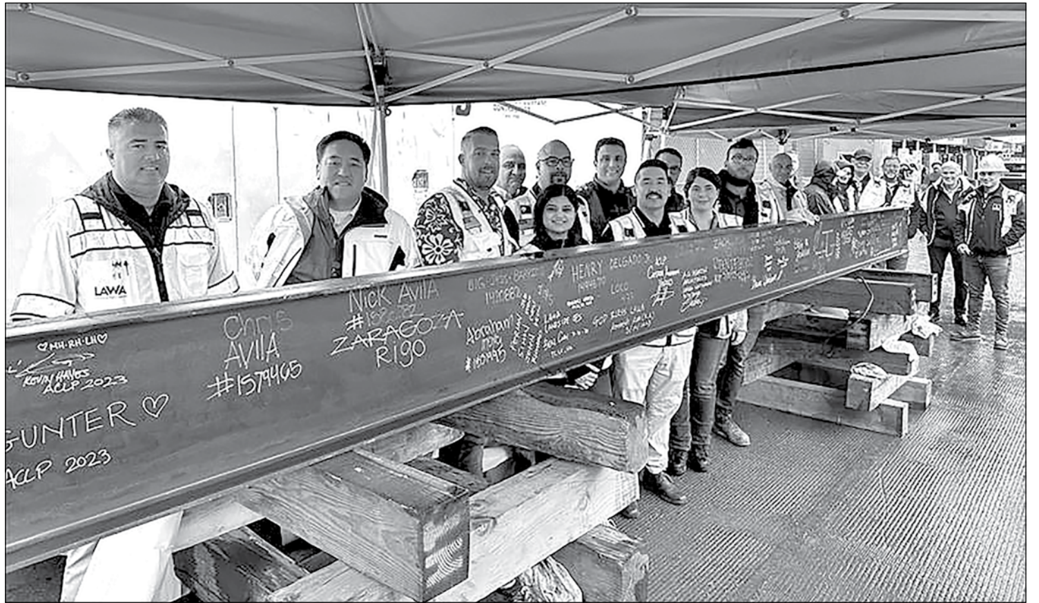
A beam signing and ceremony was held for workers of the Tom Bradley International Terminal Core. The Core is a three-level structure that will provide direct connectivity to the People Mover's West Central Terminal Area (CTA) station and is oriented for easy travel, with elevators and escalators connecting departures, arrivals, the People Mover and office spaces. In the future at this location, passengers will exit the People Mover train's pathway and be greeted by a recently restored 10-foot-tall bronze and granite sculpture memorializing the terminal's namesake, former Mayor Tom Bradley. The Tom Bradley International Terminal Core is one of seven new cores that make up the $490 million dollar Terminal Cores project at LAX, which is scheduled to complete in 2024. Photo courtesy LAX.
