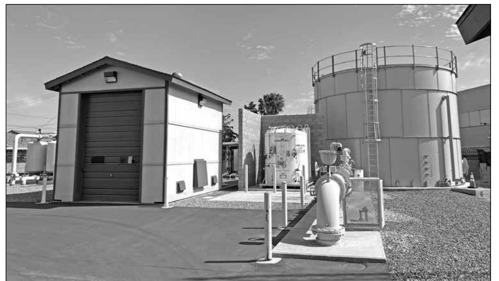
Dalton Well House and Backwash Tank.
