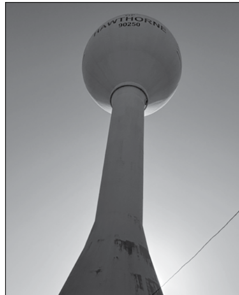
The Hawthorne Water Tower.
