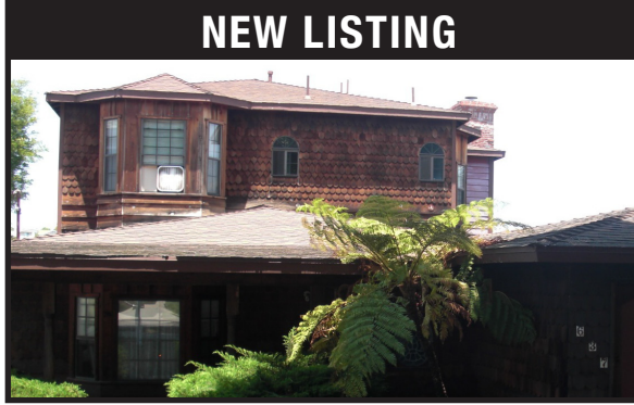
NEW LISTING 637 W. Pine — 5 bedroom, 3 bath home located in highly desirable area on a large lot.
