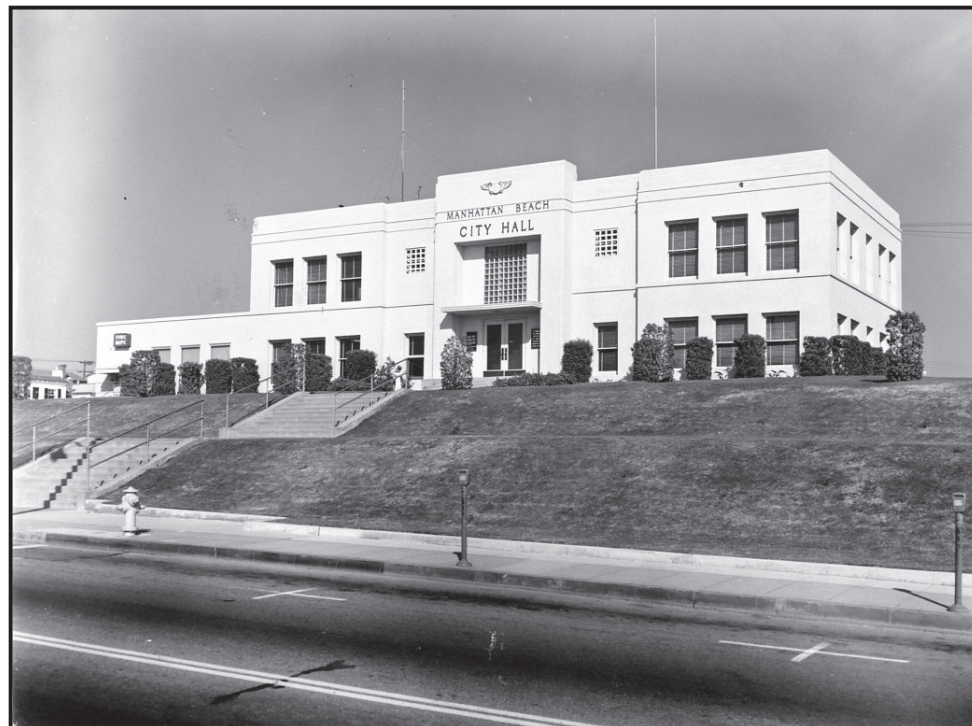
In 1937, the WPA added to the north side of the old City Hall to accommodate additional City employees.
