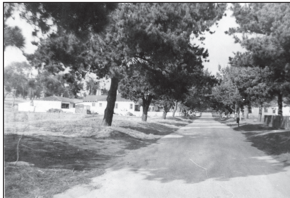
Beginning of road improvement looking north from 17th Street and Pine Avenue.
