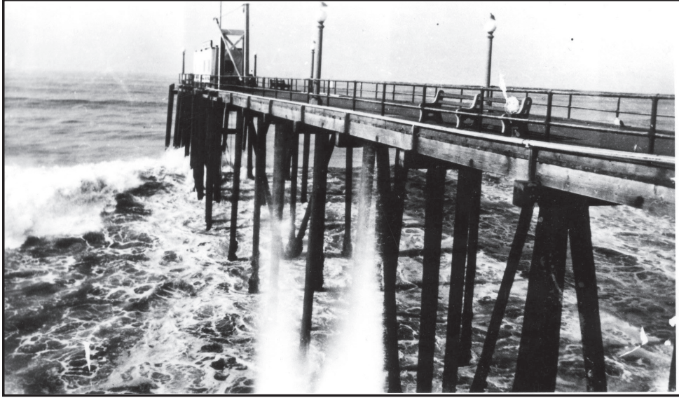
Pier extension prior to it being destroyed by high surf and strong winds. January 1940.
