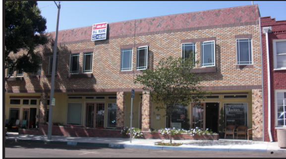
First floor retail or office space with open floor plan approx 1,210 sq ft. On second level is a living quarters with 2 bed +2 bath w/living and dining area. Private roof top deck with ocean views.
