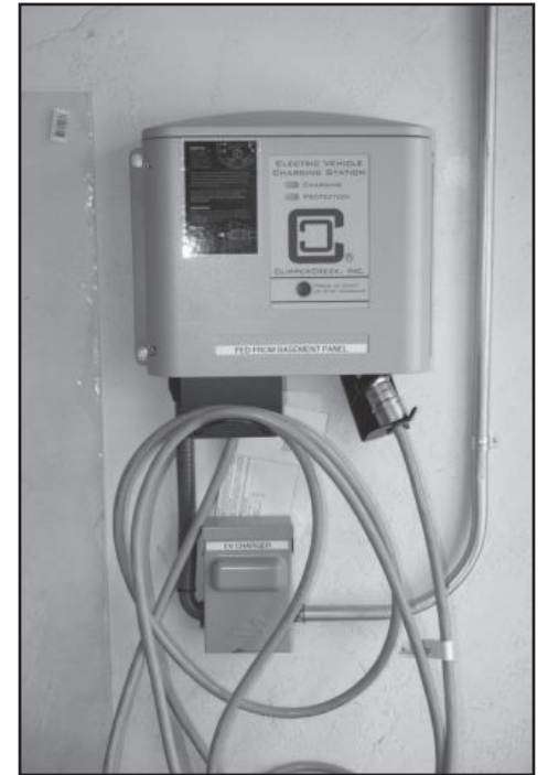
This charger box can completely recharge the MINI in less than five hours.
