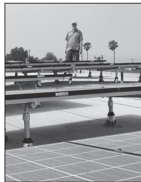
A recent solar home tour in Manhattan Beach included the Jarus home. Picture is Scott Jarus on the roof of his home with a recently installed grid-tied 7.2-kW solar energy facility using 34 photovoltaic solar panels.
