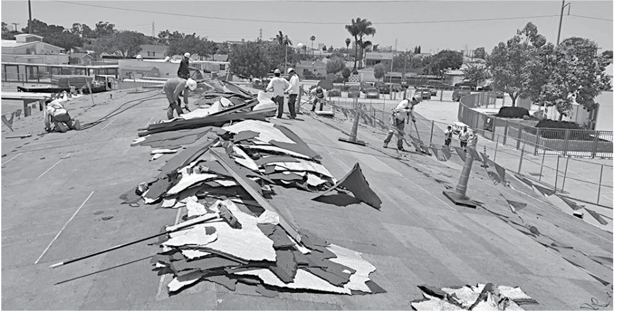
Improvements are in progress at the various Lawndale Elementary School District campuses thanks to funding from the Measure L bond passed in 2016. In this shot, crews at Jane Addams Middle School are hard at work on a new roof. Photo: Jane Addams Middle School.
