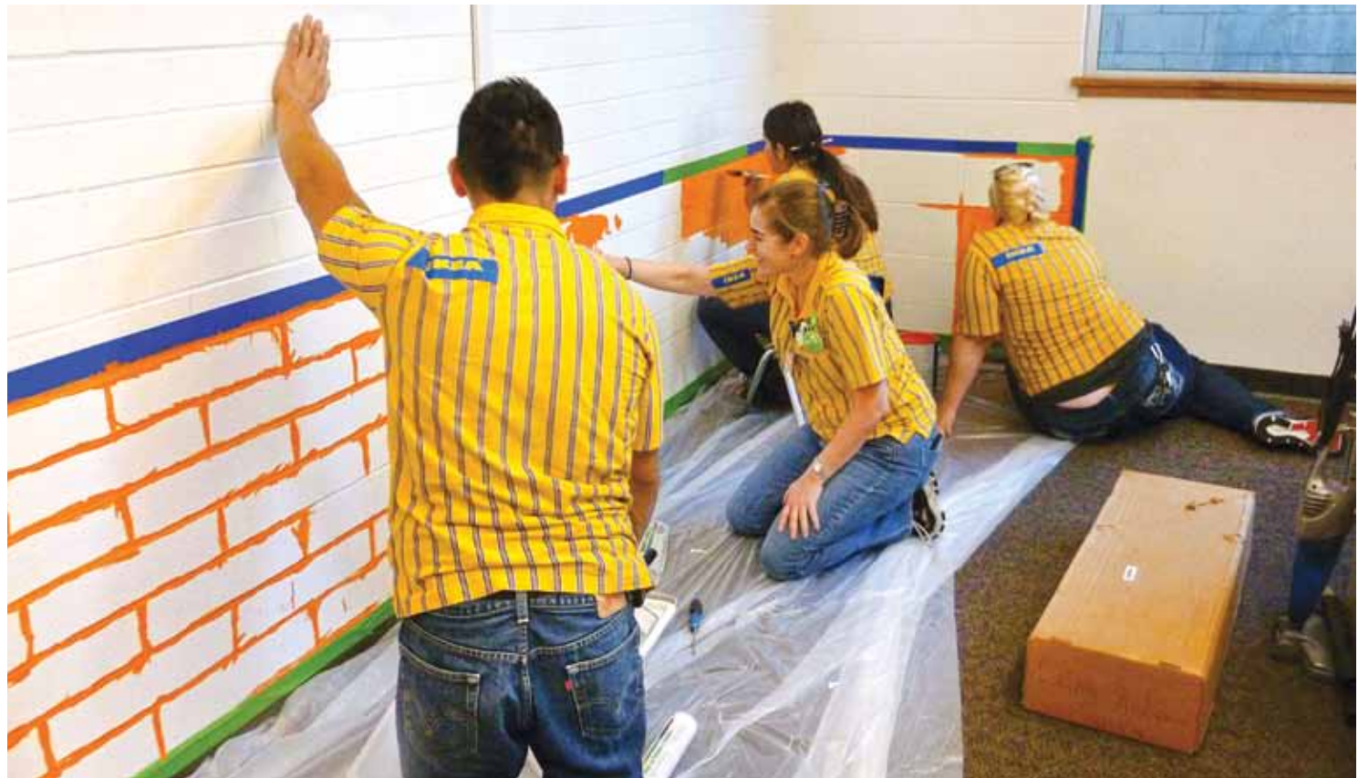
IKEA Carson employees paint cheerful walls as part of an IKEA summer remodel of the two-room library at Hickory Elementary School. The library, run entirely by the PTA, had kept books and materials on worn and crowded shelving. IKEA interior designers created functional spaces incorporating areas focusing on the needs of the younger children and the needs of older students. Workers added bright paint and soft pillows, and built new desks, chairs, bookcases and closets. Judy Nei, parent and head librarian at Hickory Elementary School stated: "Hickory Elementary and its PTA will be forever grateful for what IKEA has done to extensively upgrade our school library." Photo by Jessica Azerrad
